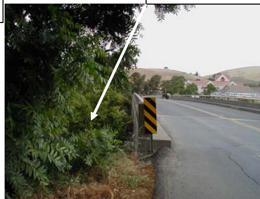
I-780 over crossing prior to improvements
